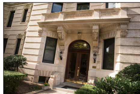
The front facade of the Mendota Apartments
