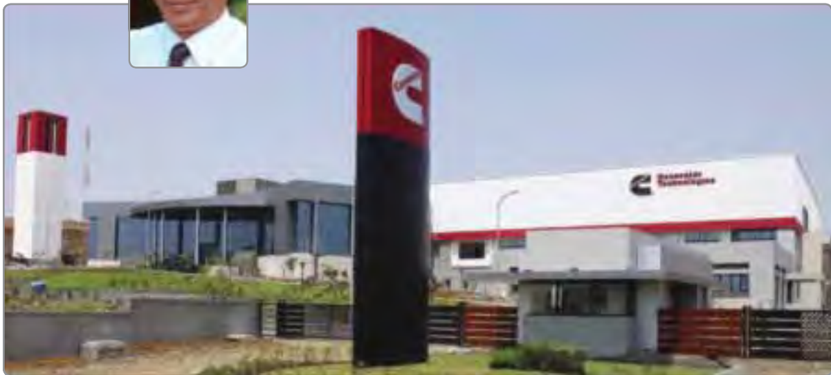
The Cummins Generator Technologies plant at Ranjangaon.
