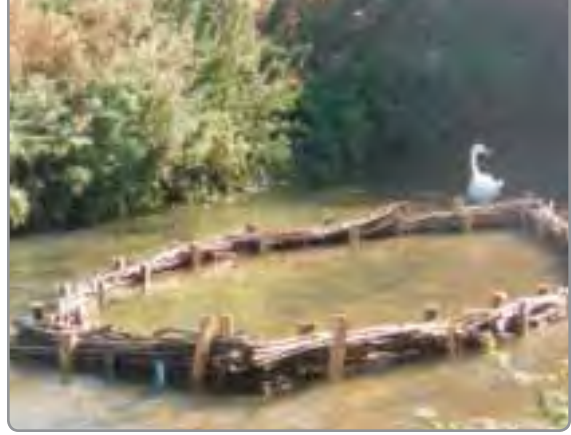
The mid-stream island begins to take shape.
