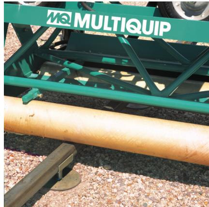
**Step 3** — Now you are ready to pour the concrete — and achieve the flattest floors ever with the SuperScreed. Using the chair and rail system, this slab measured final FF numbers of 89!
