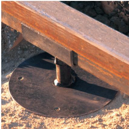
**Step 2** — Using the built-in jack system, the screed is easily placed on the rails.
