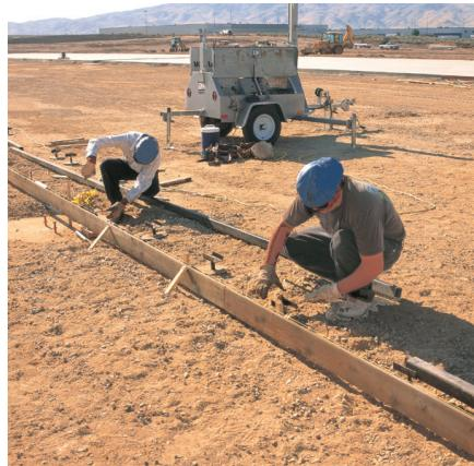
**Step 1** — Minimal forming is needed. Assembly chair and rail system using only two workers. Measure for levelness using such basic tools as a measuring tape and level.
