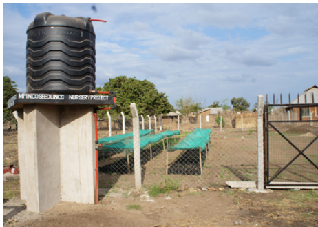
Built tree nursery facilities, such as pump, water tank, and well in corner of local agricultural village
