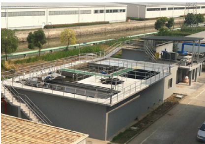
Wastewater treatment facility (Hangzhou Yamaha)
