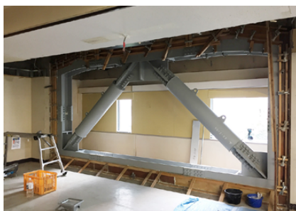
Improving earthquake resistance at a Nagoya site
