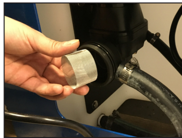
Unscrew See-through Cap (Left Photo); Remove and Inspect Filter (Right Photo)
