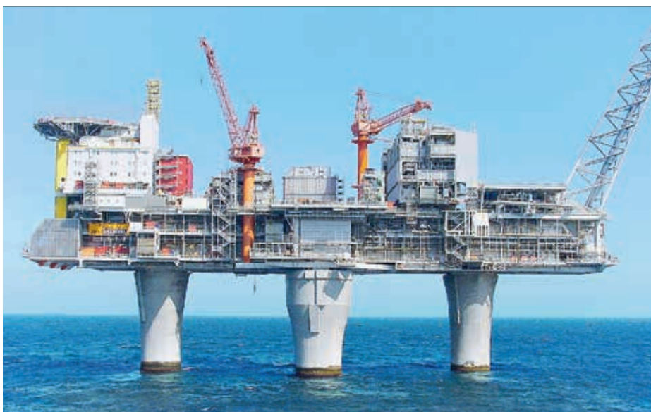
2 Troll A platform. The HVDC Light station is the gray box between the cranes.
