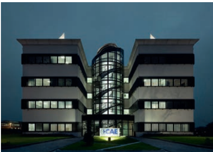
CAE headquarters in Bologna (Italy).
