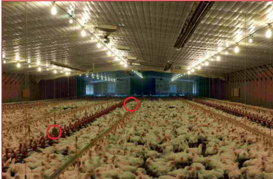
Figure 13: Correct location for temperature and humidity sensors.
