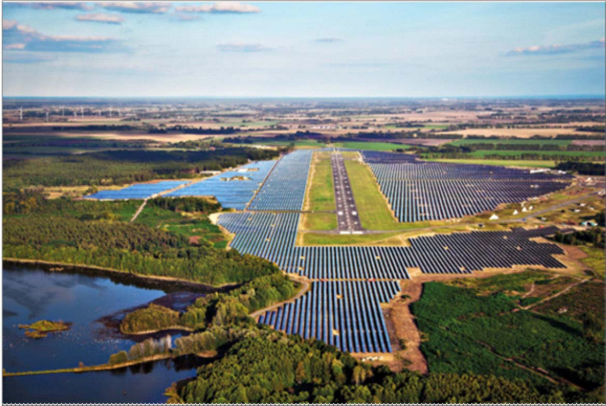
Figure 3-1. Solar power plant — Neuhardenberg Airport, Germany, 1.4 megawatt (photo source: power-technology.com)
