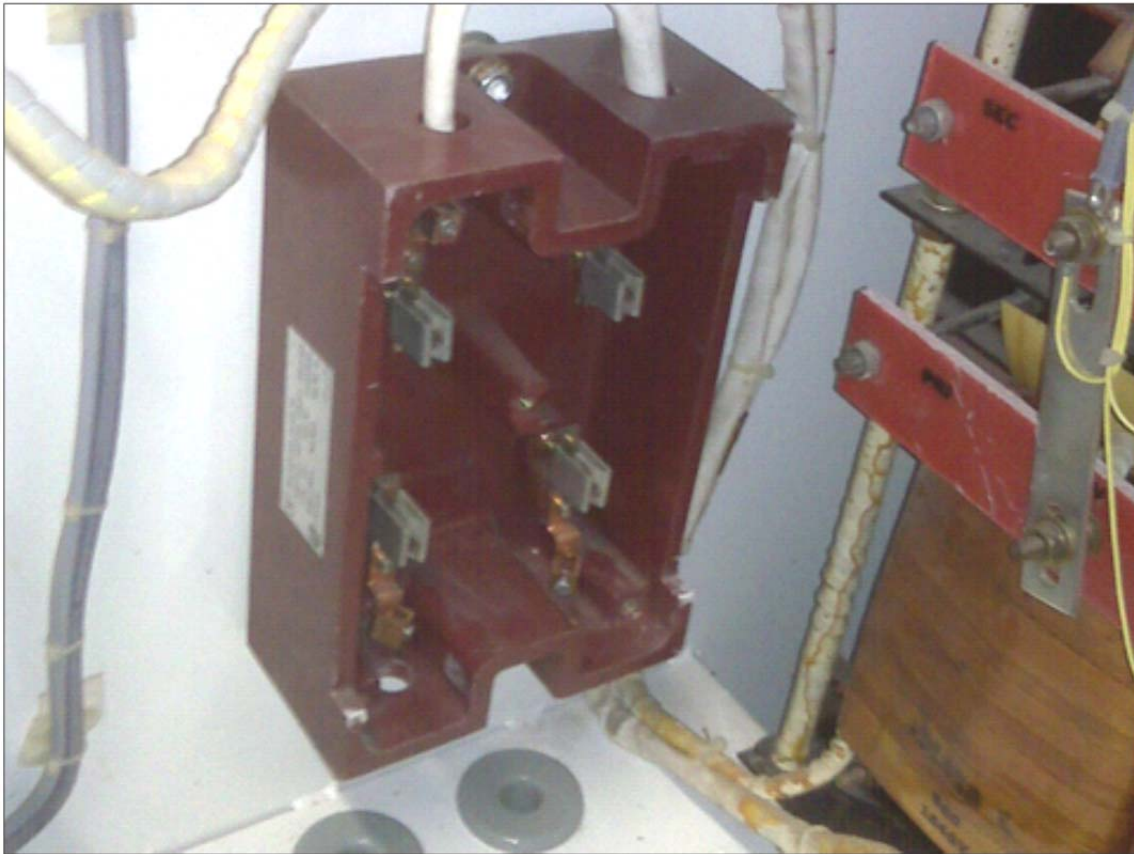
Figure 5-3. Series cut-out device receptacle (source: Liberty Airport Systems)
