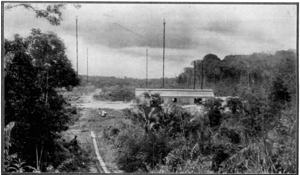
General View of Manaos Station.
