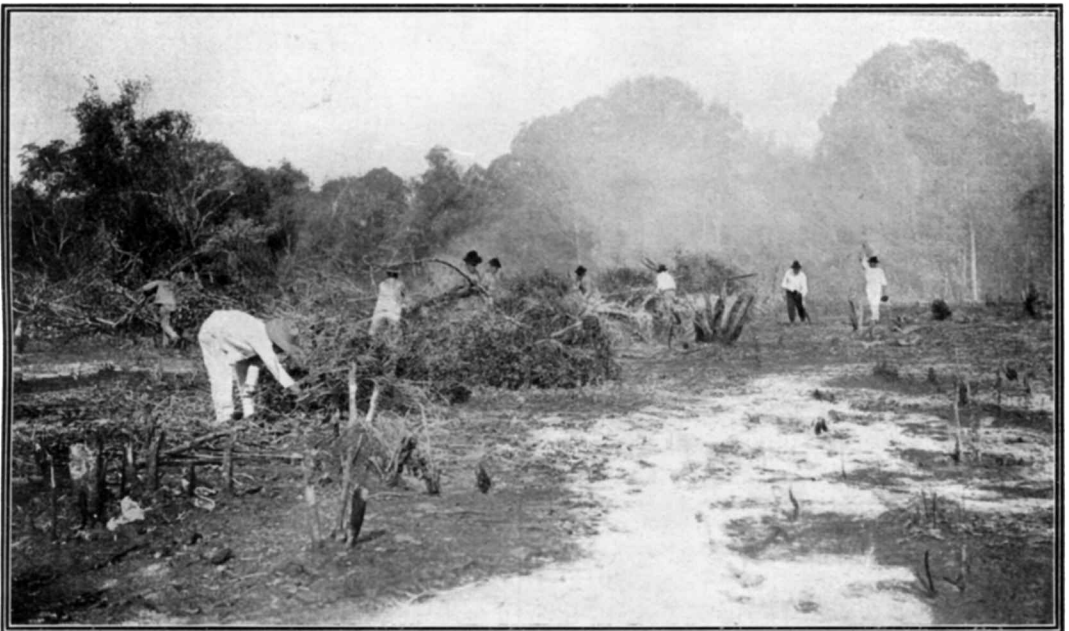
Brazilians clearing space for the Site selected for the Manaus Station.
