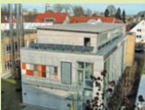
Complex G of Biberach University of applied sciences – teaching, research and demonstration building for building climate control studies and Institute for Building and Energy Systems
