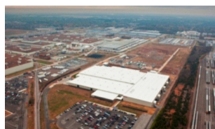
Smyrna automotive battery plant
