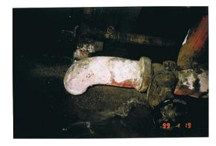
Damaged asbestos thermal insulation on pipework
