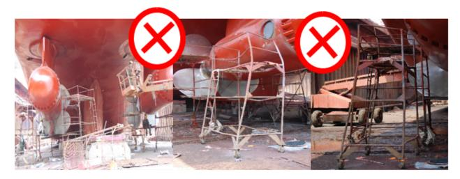
Figure 16: Damaged and dangerous mobile scaffolding
