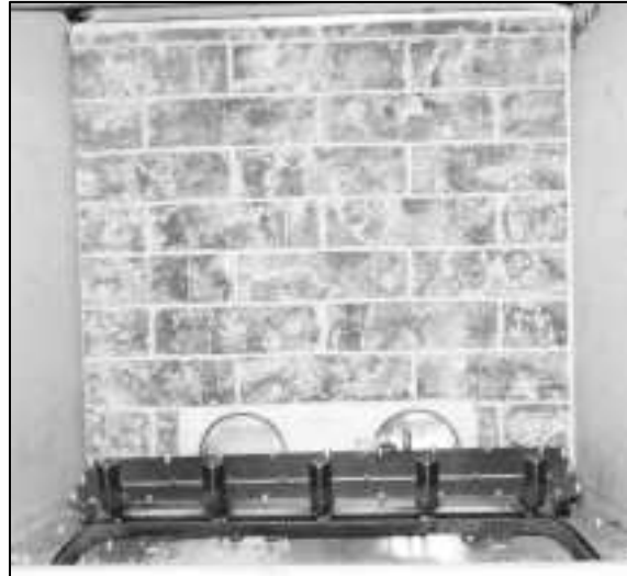
Step Two: Place Back Liner against back wall of firebox.
