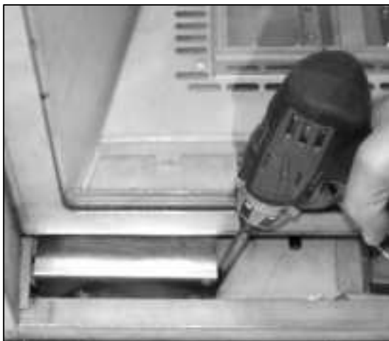
Power Vent Control Module Mounted inside fireplace.
