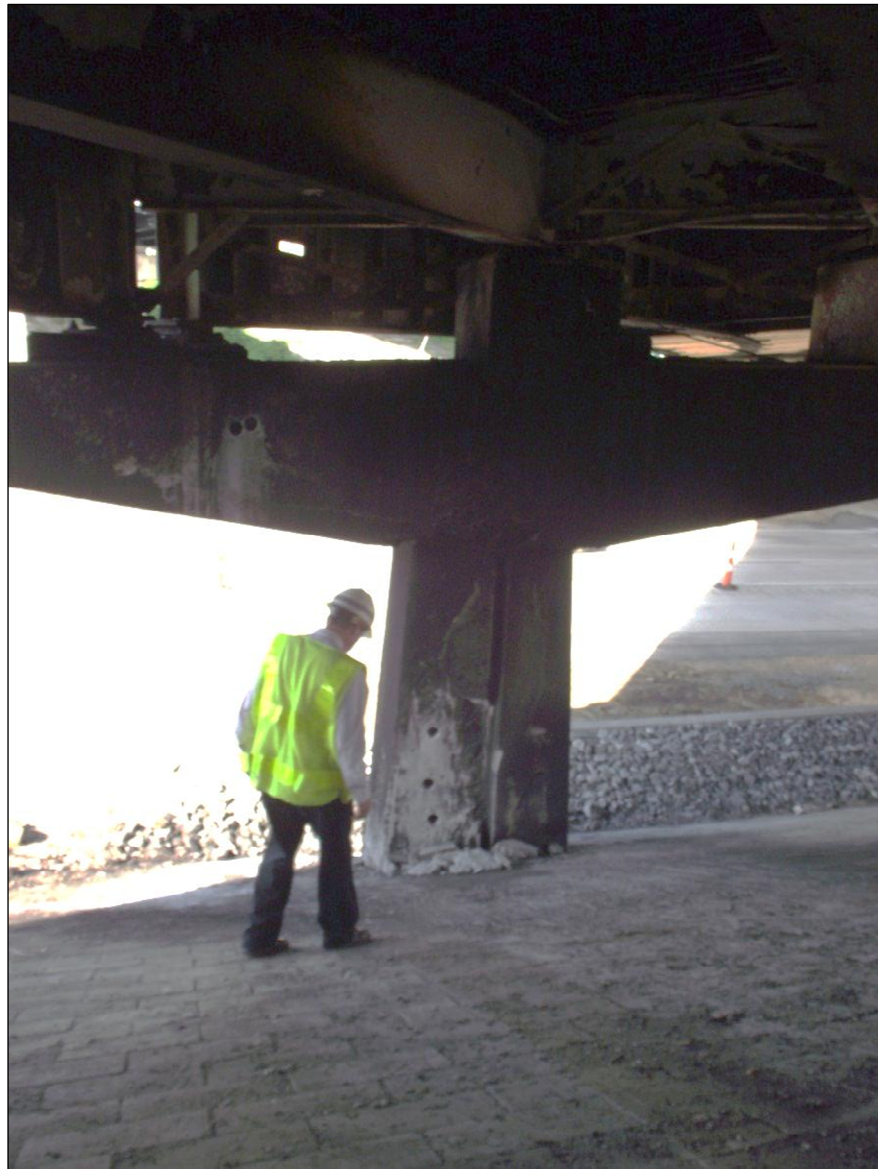
Figure 5 – Location of Concrete Cores
