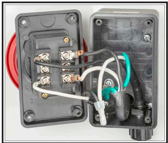
Figure 90. Cabinet E-Stop button.
