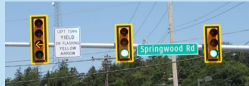
Flashing Yellow Arrow left turn phasing and retroreflective border on backplates
