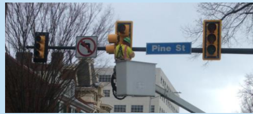
Upgrading 8" to 12" signal heads
