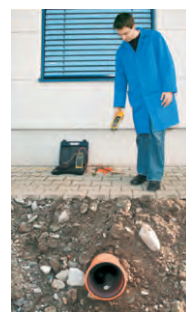
Tracing of underground cables (max. depth 2.5m)
