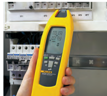
Location of fuses/breakers and assignment to circuits
