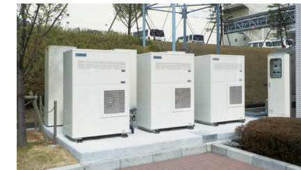
Installation of SOFC* Systems (Shiga Yokkaichi Plant, Japan) *Solid Oxide Fuel Cell
