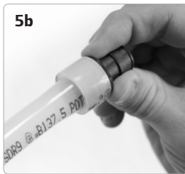
ProPEX Fitting Inserted into 1/2" Uponor PEX Tubing. Make the Fitting with a ProPEX Hand Expander Tool.
