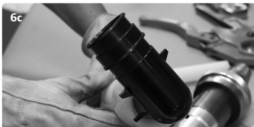
ProPEX Fitting Inserted into 2" Uponor PEX Tubing
