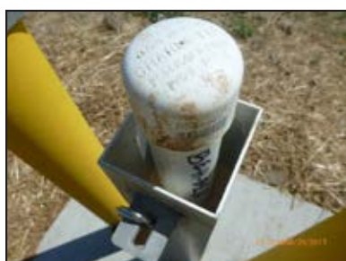
Surface protection for top of well
