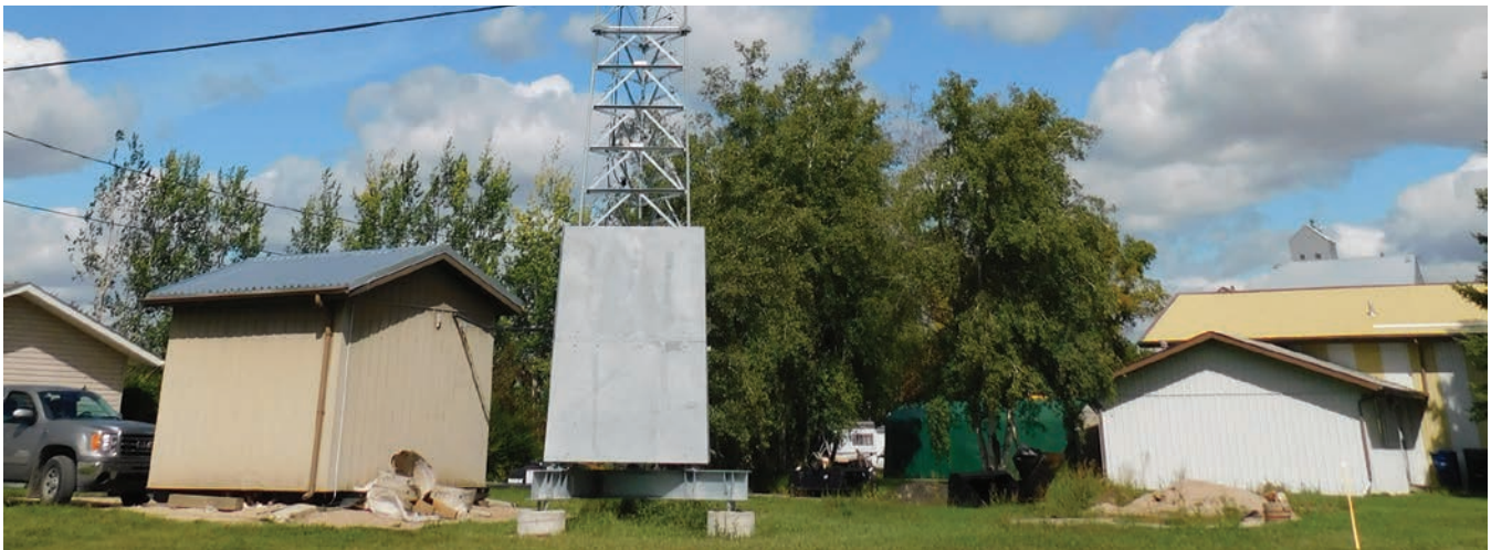
One of SaskTel's small cell sites in Bulyea, Saskatchewan.
