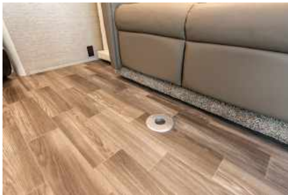
Figure 102.1 Vinyl Flooring in Living Area with Carpeted Slide Out Room Shown
