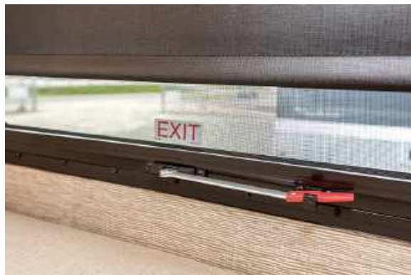
Figure 28.2 Emergency Exit Window in Bedding Area
