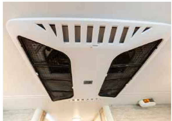
Figure 34.2 Chill Grill Covers Removed Exposing Vent Filters. Remove and Clean Periodically. Let Dry Before Reinstalling
