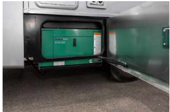
Figure 82.1 Onan 3.2kw Diesel Generator
