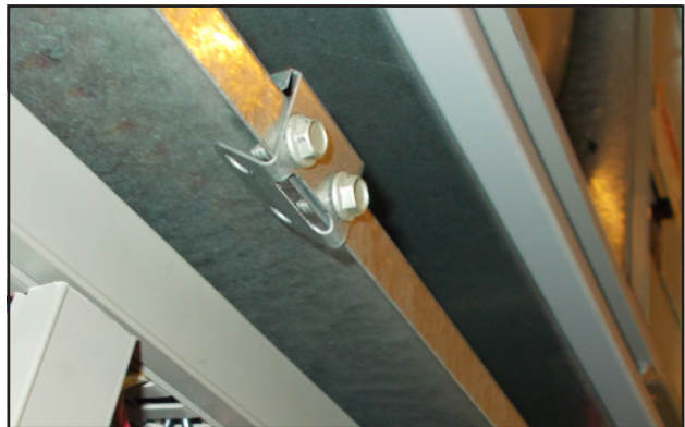
FIGURE 8 Re-Install Screws and Bend Tabs Up
