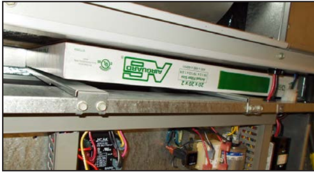
FIGURE 10 Install Left 2" Filter
