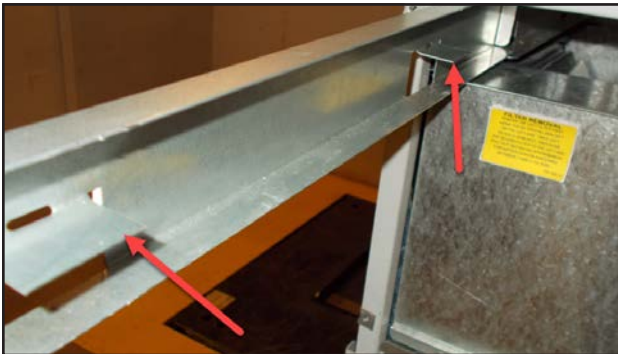
FIGURE 4 Filter Tabs in Up Position
