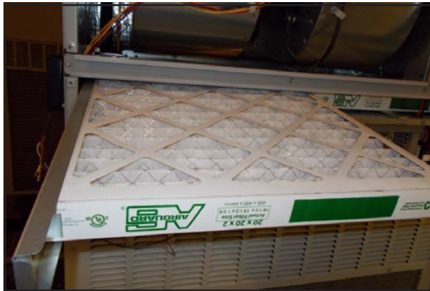
FIGURE 10 Install Left 2" Filter
