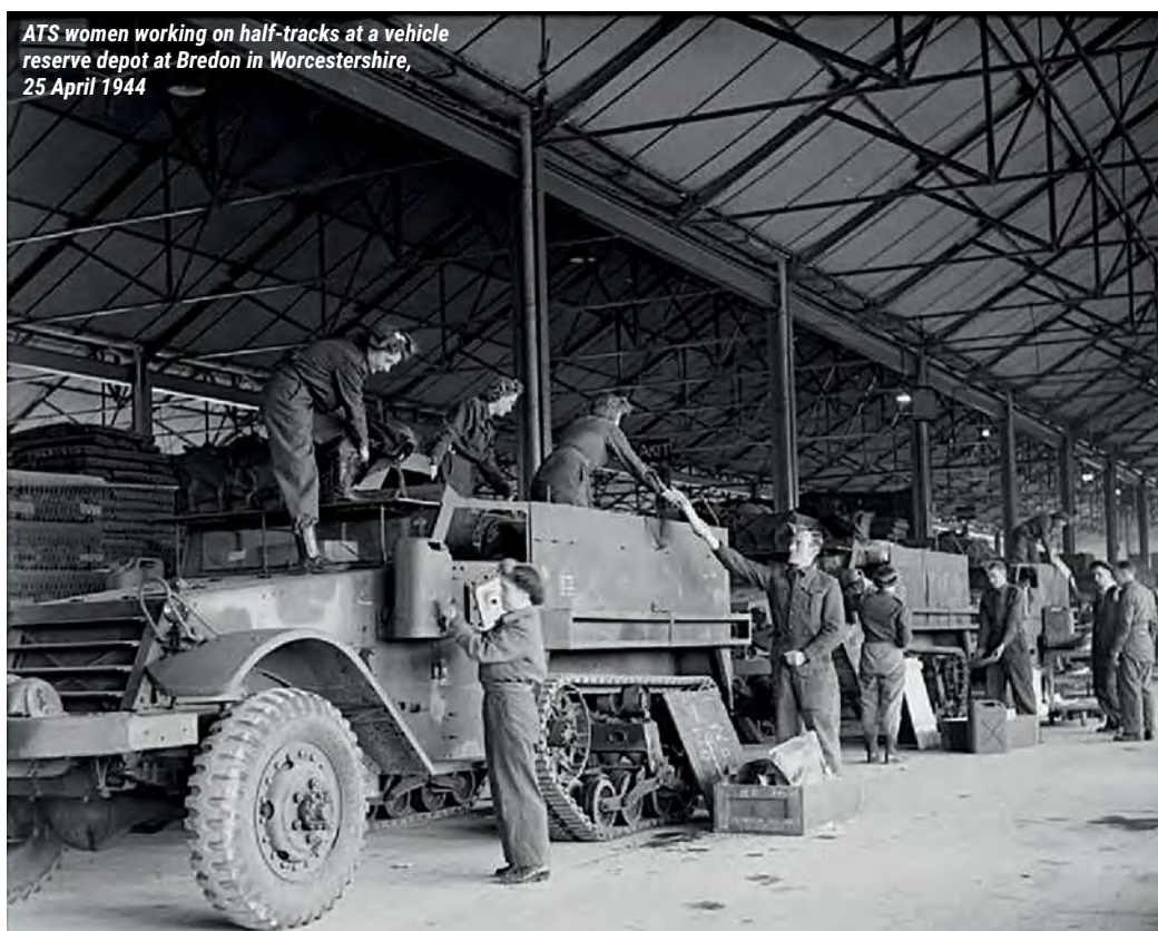
Pioneer tools were carried on each side below the cab doors, the half-track is amply fitted with externally accessible lockers, racks, boxes and hooks
