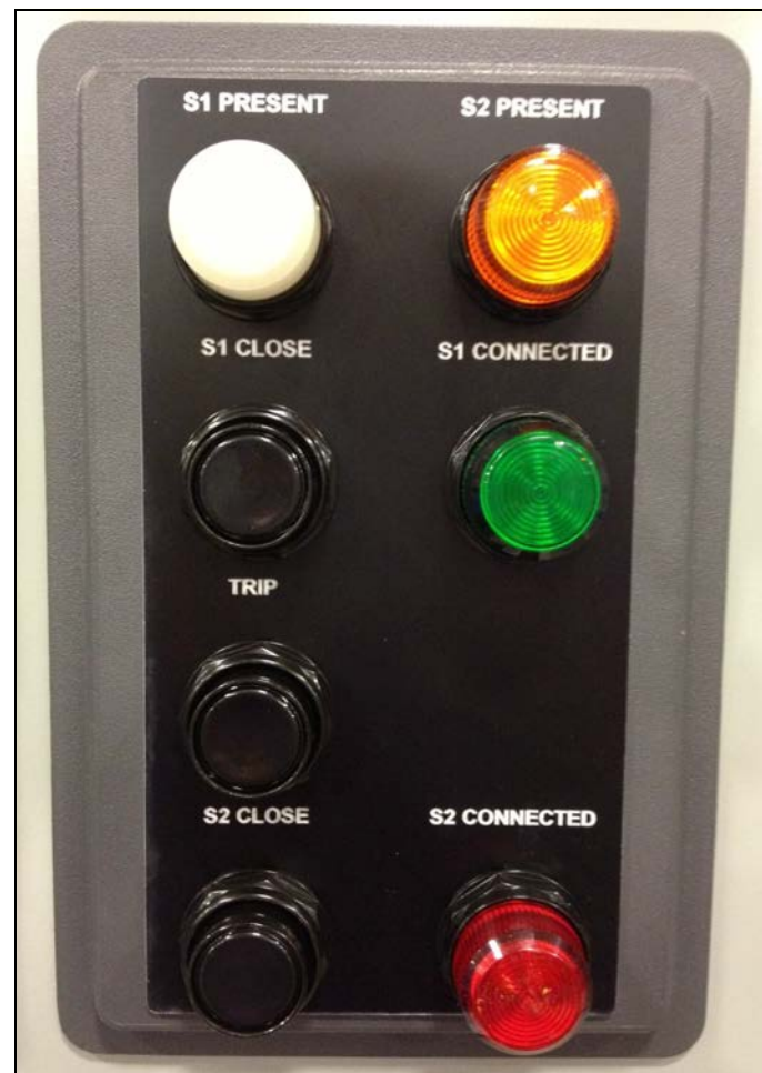
Figure 14. Non-Automatic Controls.
