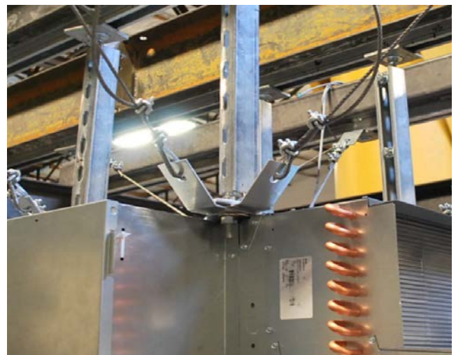
FIGURE 7 – OVERLAPPED FLAT AND 45° BRACKETS
