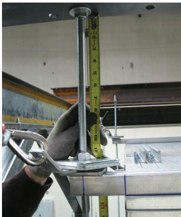
FIGURE 4 – RECOMMENDED LENGTH OF THREADED ROD
