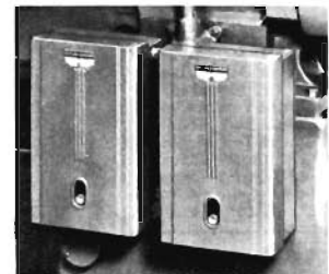
Line-starter Control Equipment for two-speed motor
