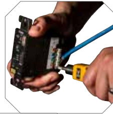
Termination Quick, reliable 110 punch down termination
