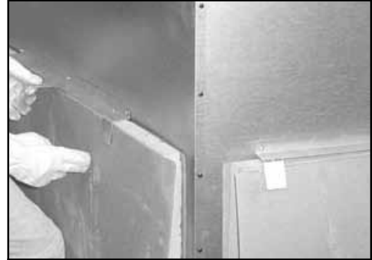
Figure 7.1 Unpacking Back Refractory
