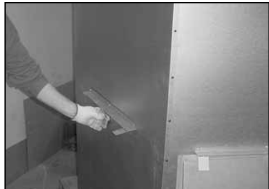
Figure 7.2 Bending Refractory Shipping Tabs Back Down
