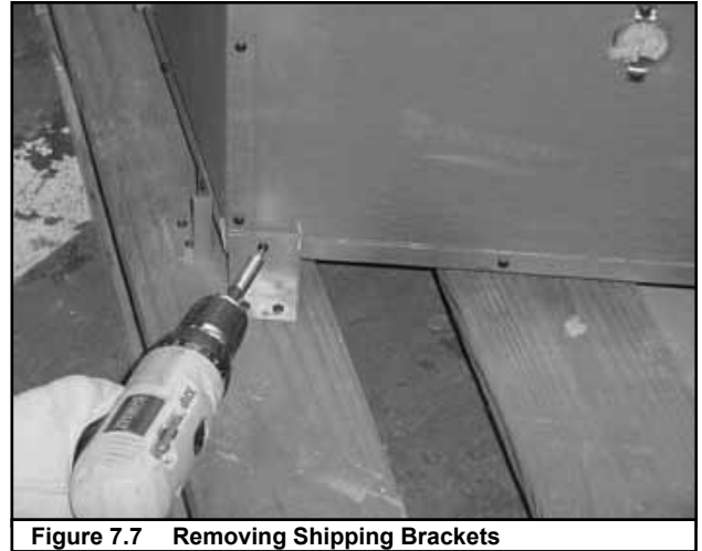
Figure 7.7 Removing Shipping Brackets
