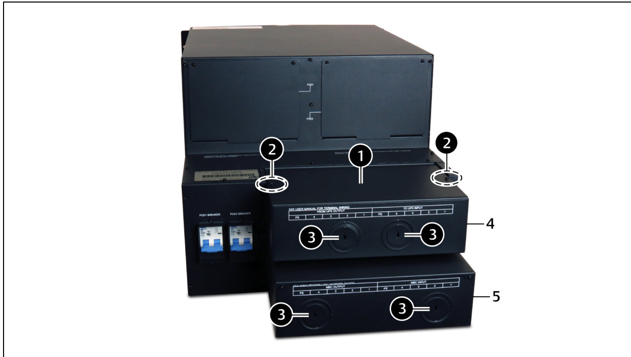
Figure 3.3 Remove the conduit boxes
