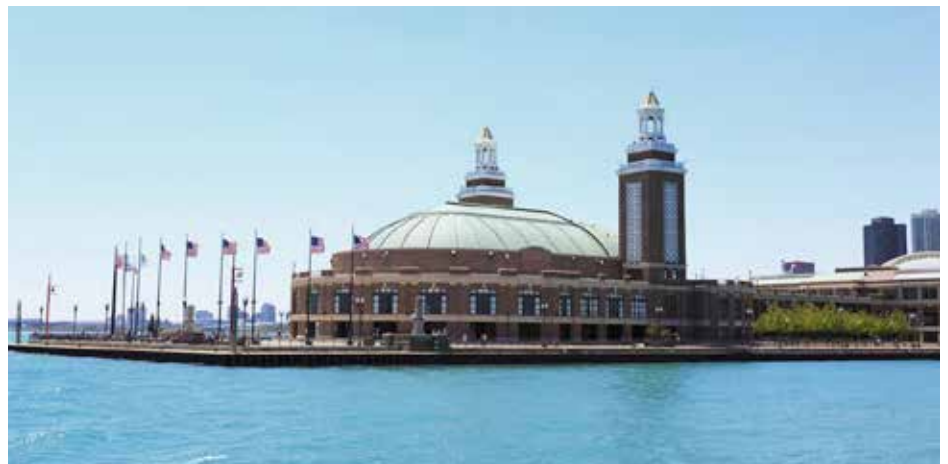
AMS used Sloan products for the Welcome Pavilion on Chicago's Navy Pier because many of the products come preassembled, which speeds up installation and saves labor costs.
