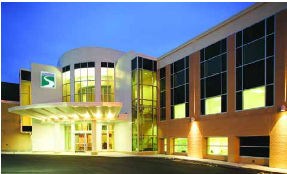
Southern New Hampshire Medical Center in Nashua chose Daikin chillers primarily for their energy efficiency but has also seen reduced maintenance costs since installation.
