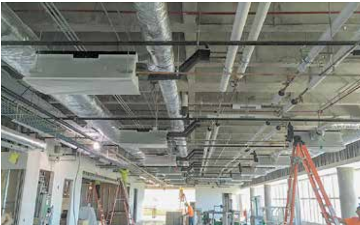
Left: To meet the tight construction schedule for Carrier's state-of-the-art headquarters, Hill York recommended setting Carrier's ActivAir chilled induction beams in place before the ceiling contractor's installation—a dramatic timesaver.
