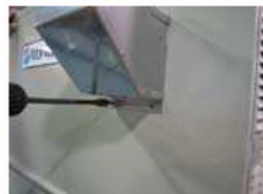
SECURE HOOD TO UNIT WITH TWO SCREWS
