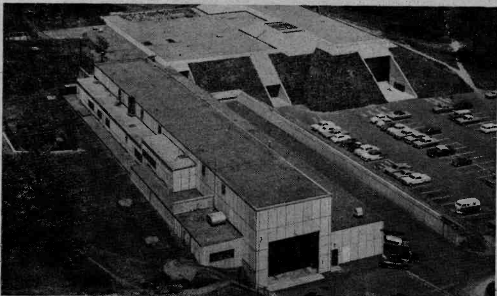
Overall view of Laboratory, looking north toward East Rock. Heavy Ion and Electron Linear Accelerator Laboratories appear at left; three entry doorways lead to storage space, offices and laboratories, and accelerator vault, respectively. Truncated pyramids on roof contain cooling towers for closed loop water supply in Lab.
