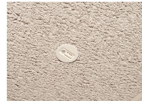
Step 4: Sensor will clamp into place. Turn sensor to appropriate position.
