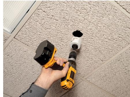
Step 1: Drill 2.5-inch hole in ceiling. It may be more practical to remove the ceiling tile and drill from the backside depending on material.
