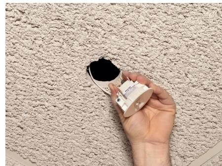
Step 3: Compress spring clips on sensor and insert into ceiling hole.
