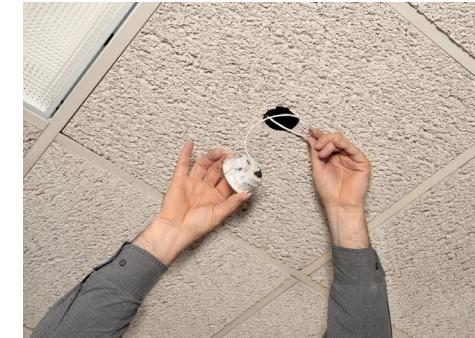
Step 2: Feed wires from sensor into ceiling hole. Wire length provided is 36-inches. Cable jacket provided is plenum-rated. Add additional wire length if necessary (18AWG solid wire recommended).
