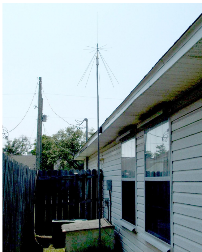
External antennas such as this one must be taken down to survive a storm threat.
