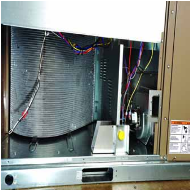
Figure 17: Flue Exhaust Hood Shipping Location
