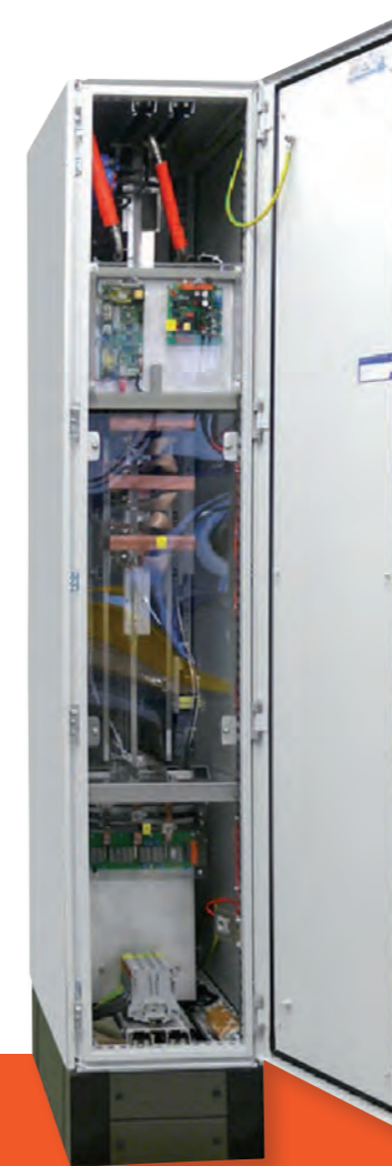
Hollow rope testing with 5000A
