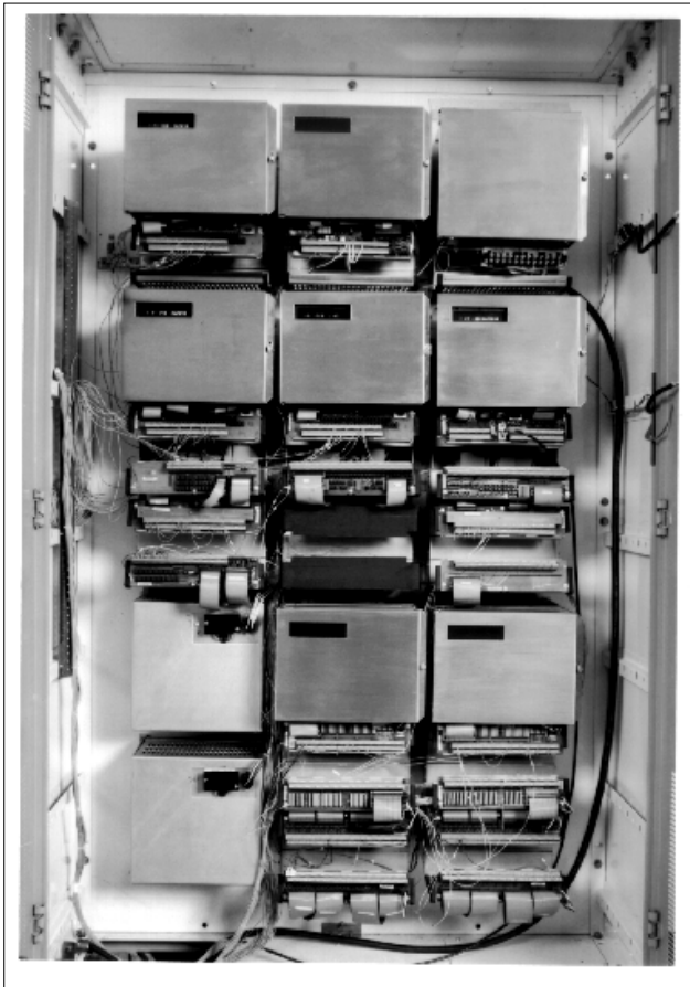
Figure 1. SPEEDTRONIC™ Mark V steam turbine control cabinet
