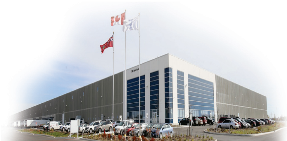
Airport Road, Brampton
