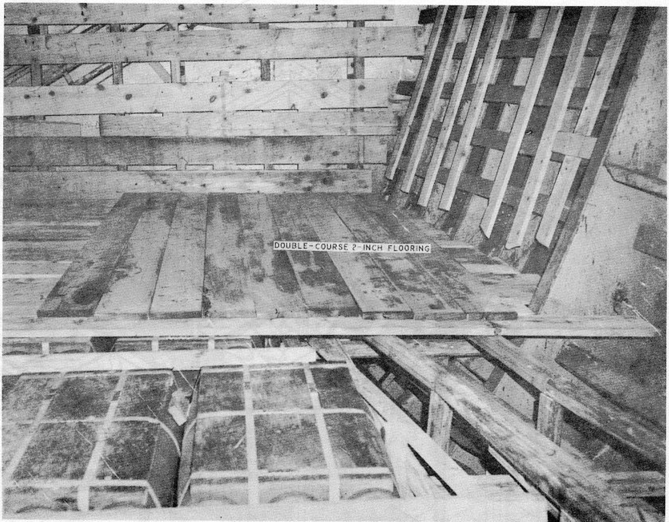
Figure 9-49. Completion of flooring prior to stowage of additional tiers of bombs (hull blocking technique).
