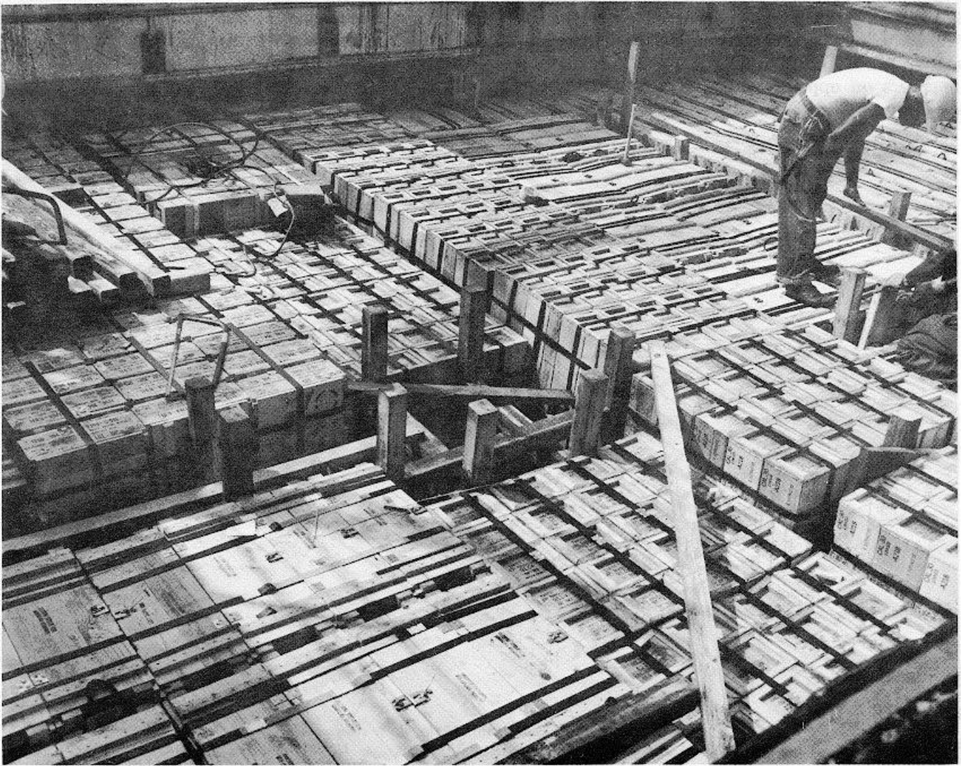
Figure 8-19. Final void shoring in progress.
