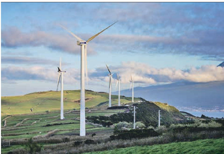
4 Wind-diesel microgrid on the island of Faial, in the Azores
