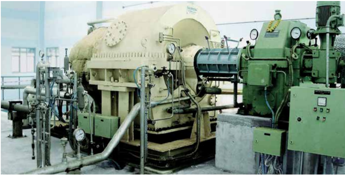
Roi Et, Thailand: Turboset for the Bua Sommai Electricity biomass power plant.
