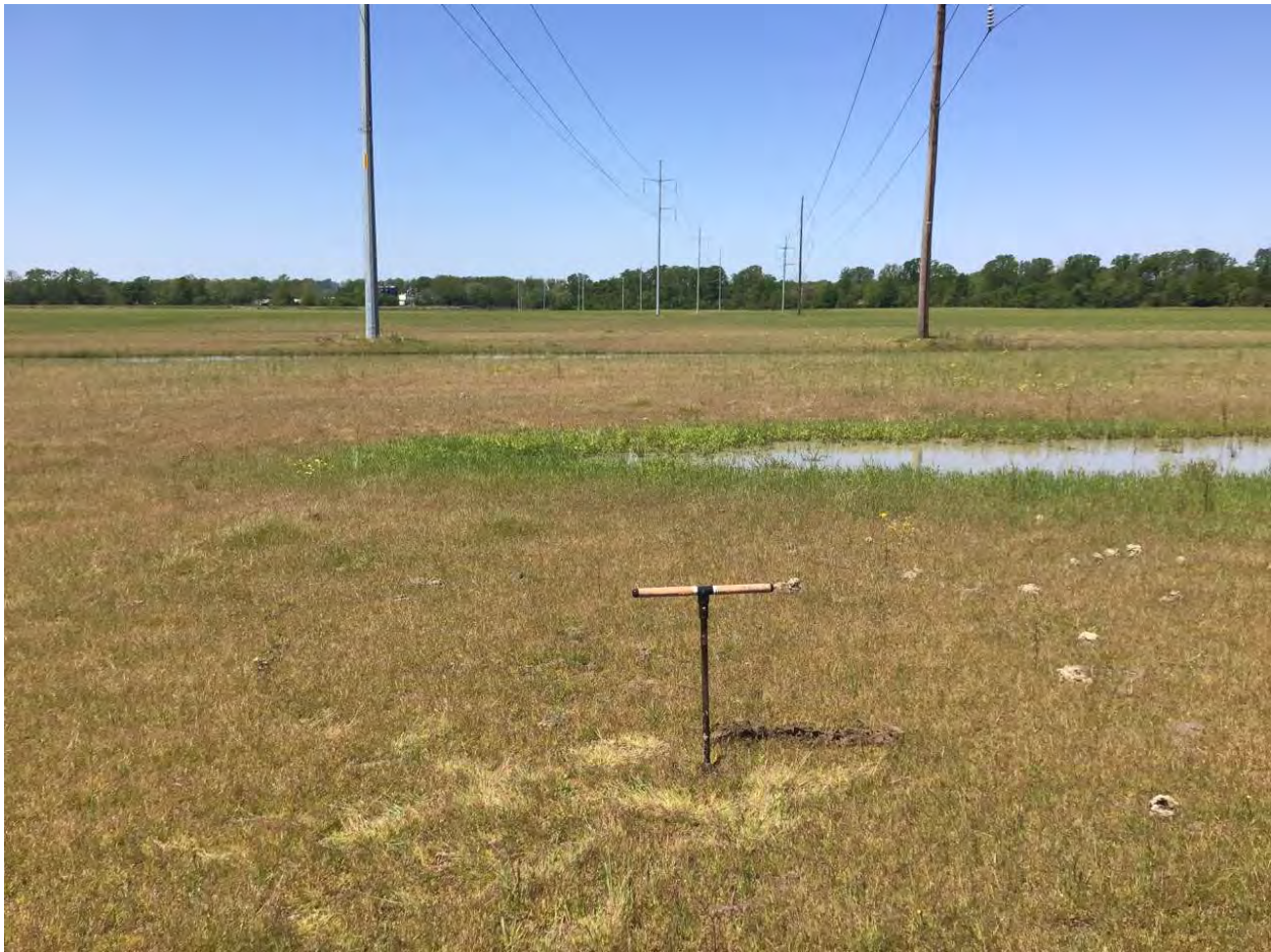
Figure 3-9: Representative Photo of Weakly to Union City 161-kV Transmission Line (Weakly County)
