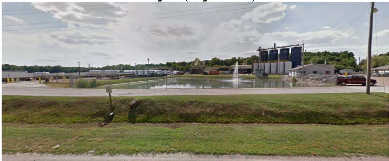
Figure 3-8: Meat Rendering Plant on Hwy 431, looking south (Google Streetview)
