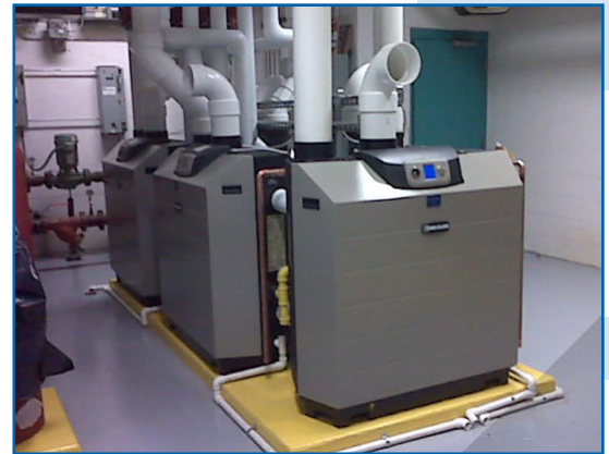
Nine SlimFit 750 boilers installed in the USARC boiler room
