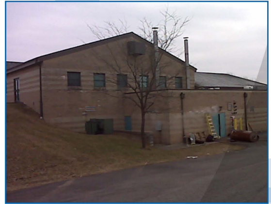
US Army Reserve Center in Morgantown, WV
