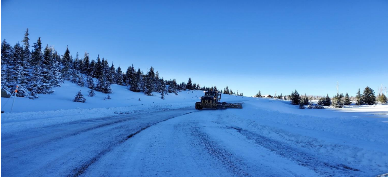
Operators benching snow with the grader wing up in Steam Engine Meadows
