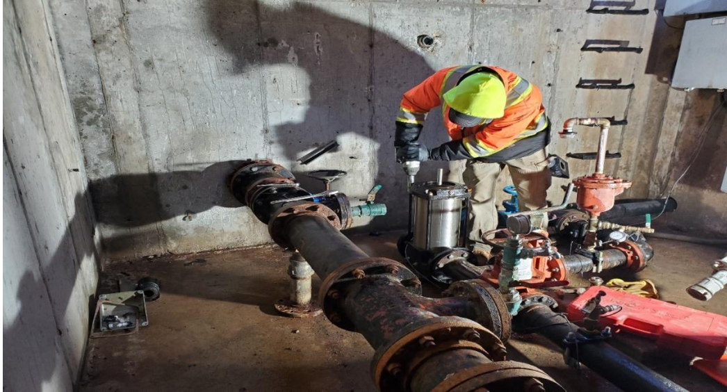
Jason Wallis re-assembling the bowl stack of a pump after inspection at the Snowflake Booster
