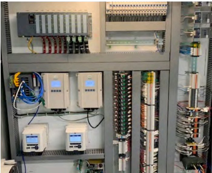
HydroRanger 200 HMI is an ultrasonic level controller that provides control, differential control, and open channel flow monitoring.
