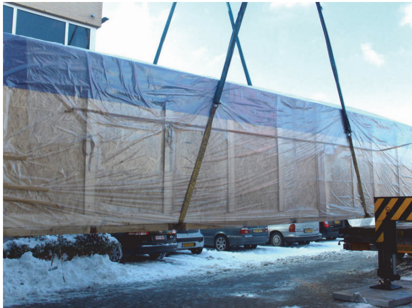
Figure 1-20 Lifting the Crate with the Heavy Crane
