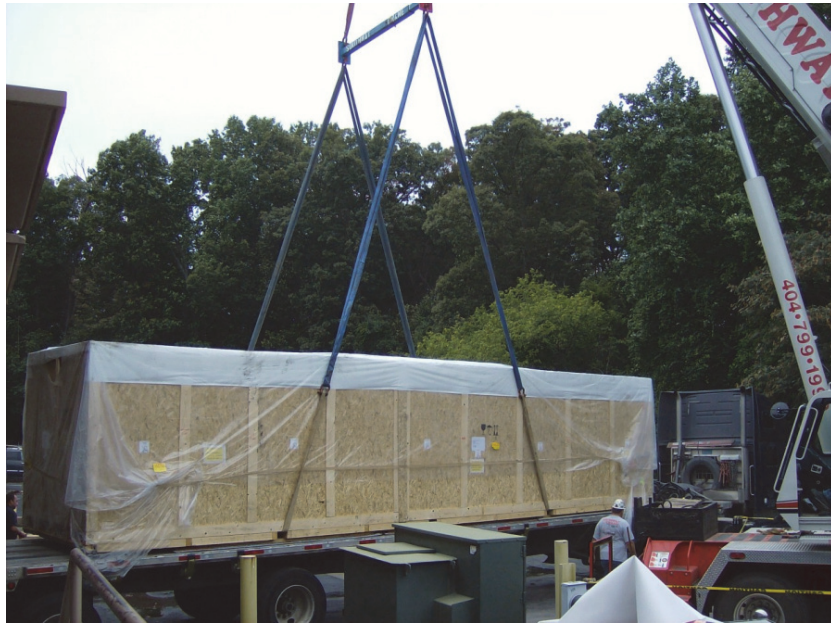
Figure 1-19 Crane Ready to be Lifted
