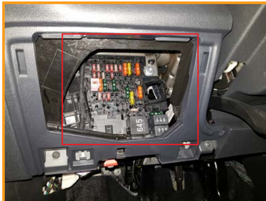
SC Relay Panel and Fuse Panel
