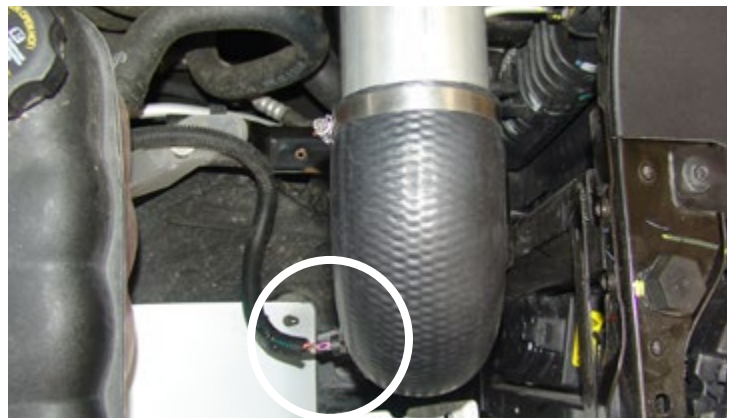
MAF Electrical Connection
